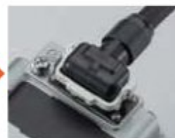
Connection is completed.
